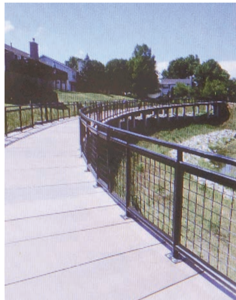
Example of a trail section with a boardwalk and railings.
