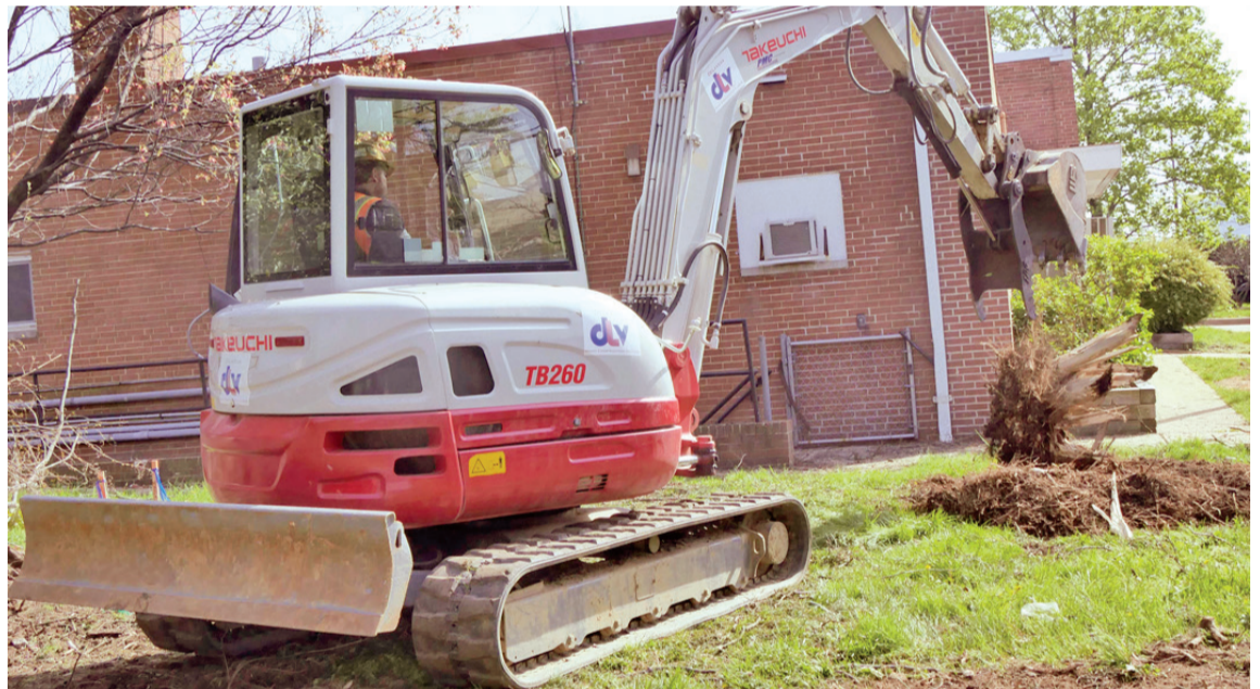
Demolition of fire station number 8 began in April 2022.
