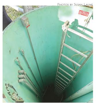
Deep below, sewage under pressure is flowing to the station's tank to be pumped to the next high point, so gravity can assist the movement toward the treatment plant
