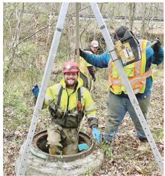
Hundreds of miles of sewer pipes are inspected annually with cameras, sensors, and lasers to assess pipe condition, sometimes requiring entry into the system to retrieve entangled equipment
