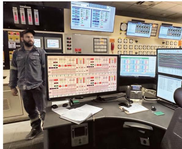
In a control room reminiscent of NASA or a futuristic starship, technicians constantly monitor process flows, combustion temperatures, and pollution control equipment and assure emissions of cooled gases released through the stack stay within or below state and federal emission standards.
