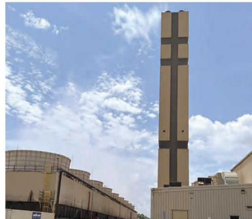
Cooling towers, on the left, expose water to ambient air after its use to cool furnaces that reach temperatures near 2,000 degrees Fahrenheit; some water evaporates and appears as clouds, most is recirculated to the power plant's condenser. Emissions stack, on right, releases cleaned gases generated after lime, carbon, and fabric filter out acid-forming gases and particulate matter
