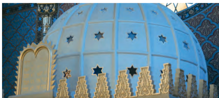
Interior of the renovated Rumbach Synagogue in Budapest, Hungary.
