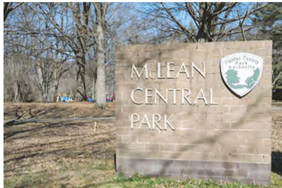
A project at McLean Central Park includes removal and replacement of walkways and playgrounds, and the addition of a new pavilion.
