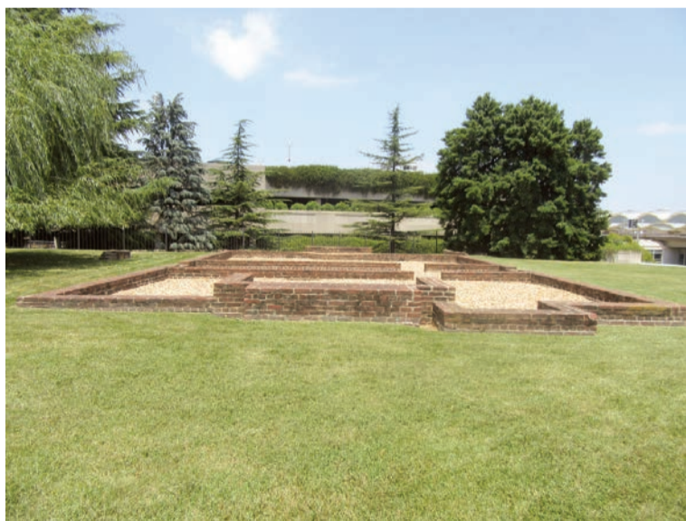
The remaining foundation of the house in the shadow of the airport terminals.
