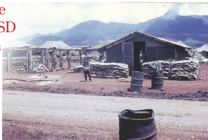
A local villager who was hired to do laundry and clean around the base at Khe Sanh.
