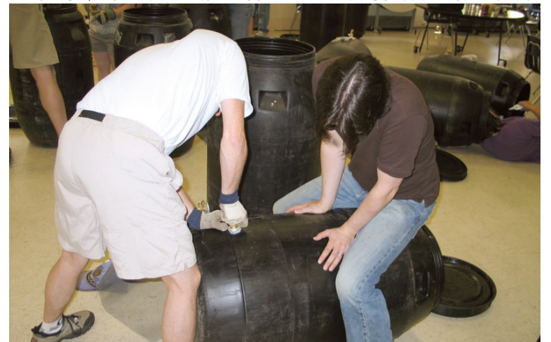
Participants at a Northern Virginia Soil and Water Conservation District Build-Your-Own-Rain Barrel Workshop glue the rain barrel’s spigot in place.
