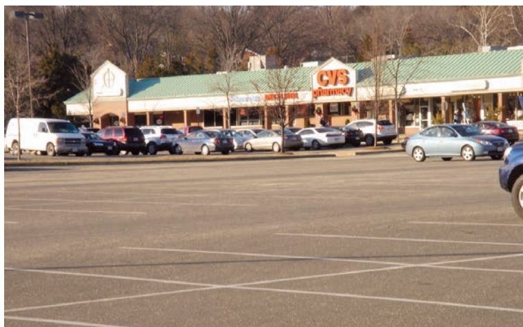
Stormwater runs off hard surfaces like this Belle View Shopping Center parking lot and pollutes area waters.
