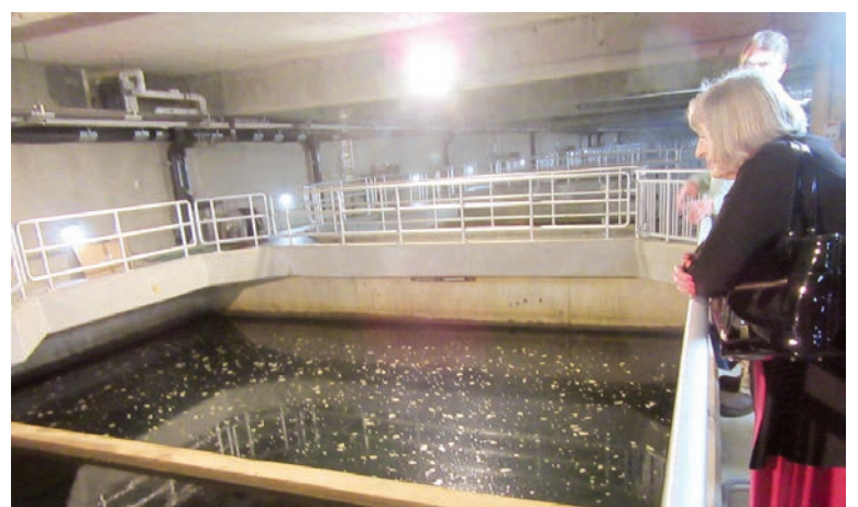
Fairfax Water treats 170 million gallons of water daily at its Lorton-area facility.
