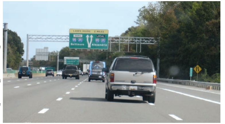
Would more toll lanes relieve traffic along this section of the Beltway that 200,000 vehicles travel daily?
