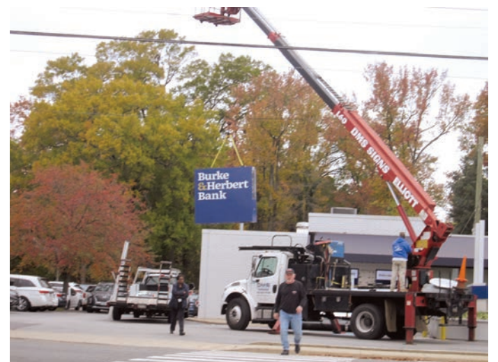
Workers installed a new sign at the Sherwood Hall Burke and Herbert bank branch on Oct. 26.
