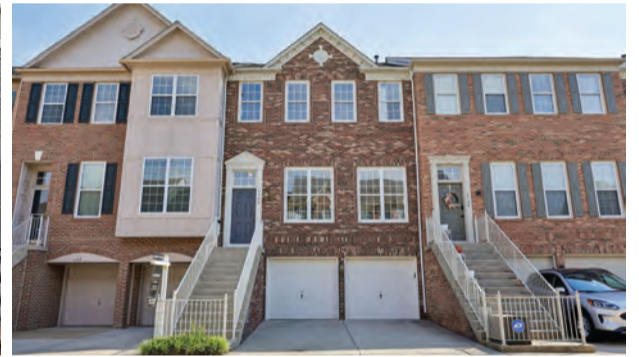
Kingstowne 6140 Manchester Park Circle
