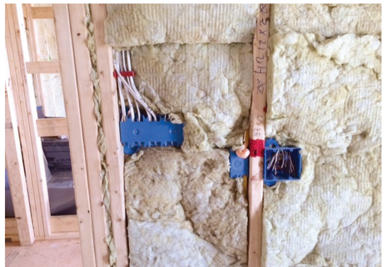
Rockwool interior insulation is in the ceilings, attic, many interior walls and under the basement slab. This also adds soundproofing.
